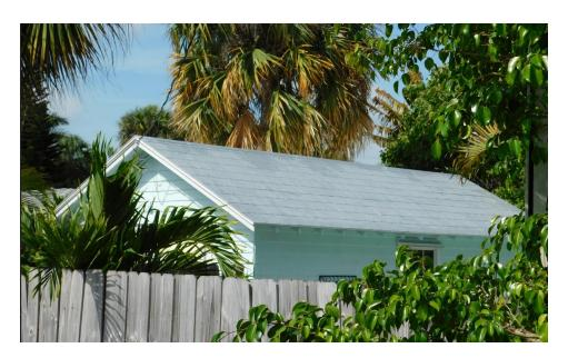
Although grey or mill finishes were most common amongst historic metal shingle roofing systems, there are also examples of metal panel systems from the 1920's on Mediterranean Revival and Mission Revival buildings that were designed to replicate a barrel tile. These metal panel systems were designed with a "pan and barrel" profile, with deep vertical channels and staggered rounded arches meant to simulate
